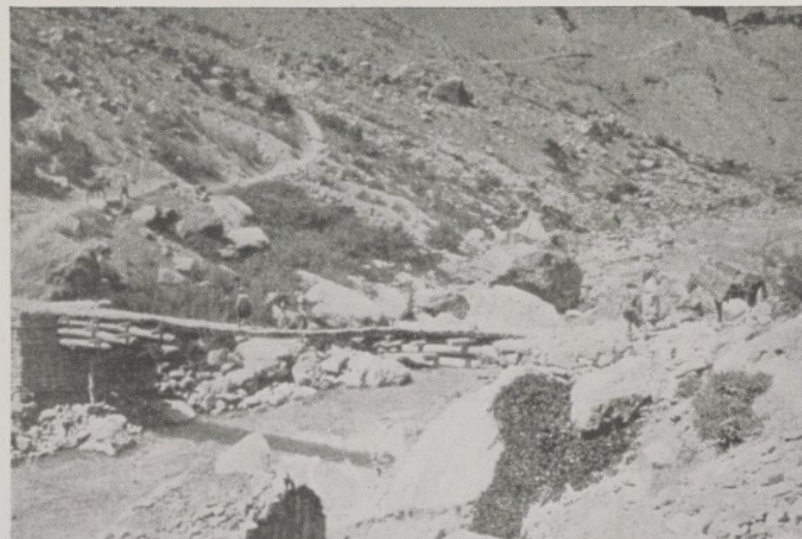
TYPICAL BRIDGE ON BAULKS NEAR JULĀMERK
